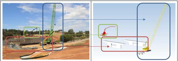
Figure 4. Comparison of a Site Photographs and As Built 4D Model on a Specified Day.
